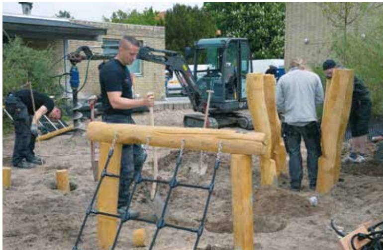
Renovering i gang, 2015.
